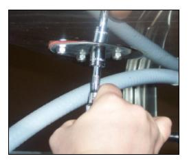
Removing the rinse drain plug
